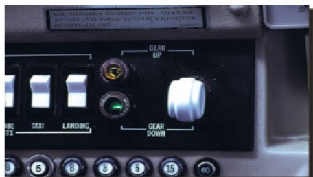
Typical landing gear switches and position indicators.
